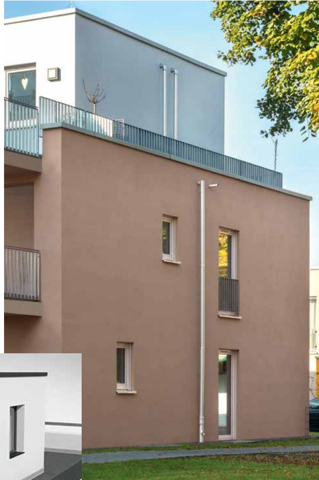
Cascade drainage – Residential complex in Duisburg-Rumeln
